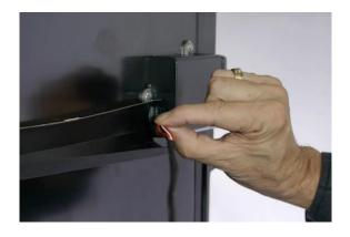
15. Drill through the 1<sup>st</sup> opening of the front grill, 8¼ inches from the right edge. This hole should be large enough to fit a finger to reach the test button.
